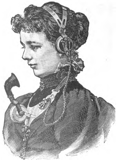
FIG. 128.—Ericsson's Breastplate Transmitter for a Switchboard Operator.
