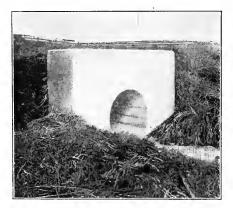
Fig. 63. A good outlet protection for a tile drain. It is desirable, however, that grating or bars be placed across the outlet to keep out and an apron upon small animals.
