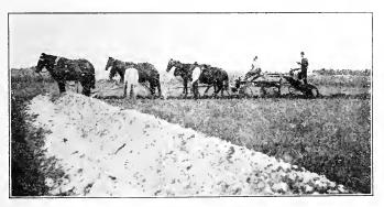
Fig. 62. Filling the ditch with a road grader.
