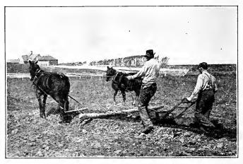
Fig. 61. Filling the ditch with a plow.
