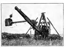
Fig. 66. A floating dredge for digging open ditches.
