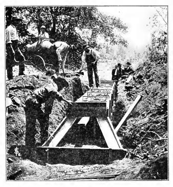
Fig. 95. Making a concrete culvert.
