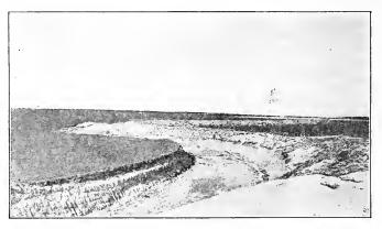
Fig. 68. Riverside Canal in Colorado before the water was turned in for the first time. This canal where shown is 18 feet wide at the bottom.
