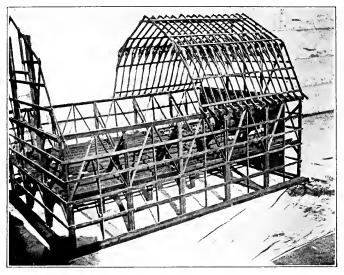
Fig. 287. A model Wing joist barn frame.
