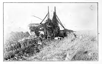
Fig. 55. A large tile ditching machine at work.
