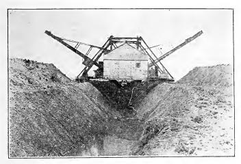
An excavator for digging open ditches, which is carried on Fig. 67. tracks laid at each side of the ditch.
