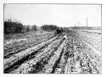
Fig. \$1. A typical condition of an earth road on which the drag has not been used.
