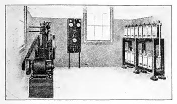
Fig. 318. Engine, dynamo, storage battery, and switchboard of an electric lighting plant.
