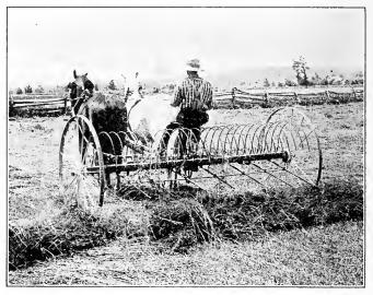
Fig. 165. A modern self-dump sulky rake at work,
