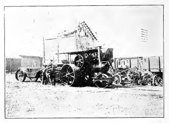
Fig. 93. Stone crushing plant. A three-wheeled steam roller and a dump wagon are shown in the foreground.
