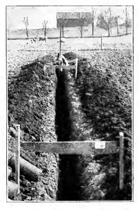
Fig. 57. The target method of grading tile ditches.
