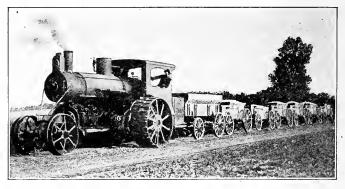
Fig. 251. An undermounted double-cylinder steam tractor.
