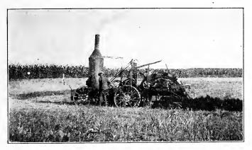
Fig. 54. A tile ditching machine at work.
