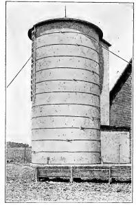
Fig. 294. A good stave silo well anchored.
