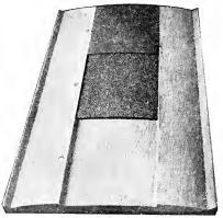
banks are provided at Fig. 83. Model of a gravel road illusthe side which will hold A shows prepared sub-grade: B, first course the gravel on the road of gravel; C, upper course of gravel. (Bul. 36, Office of Public Roads, U. S. Dept. of proper In trench conp A gr.)
