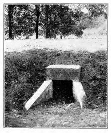
Fig. 97. Concrete culvert after the plan of Fig. 88.
